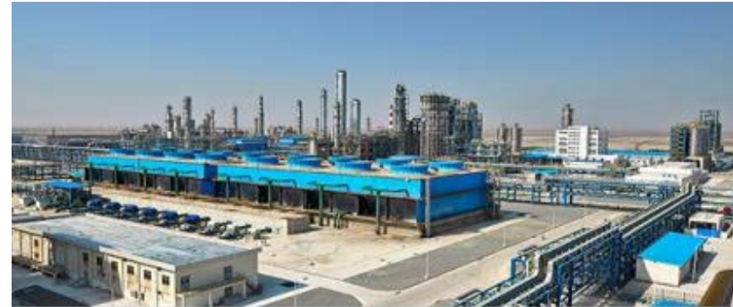
Fund Energy Ningbo 's 1.8 MMT merchant methanol to 0.6 MMT olefins plant
