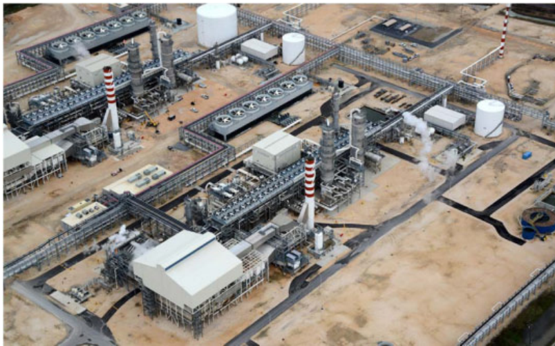
Completed Geismar 2 plant in operation*
