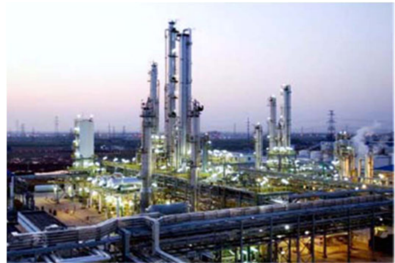
Nanjing Wison's 0.8 MMT merchant methanol to 0.3 MMT olefins plant
