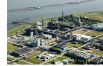
BioMCN , Delfzijl, Netherlands
